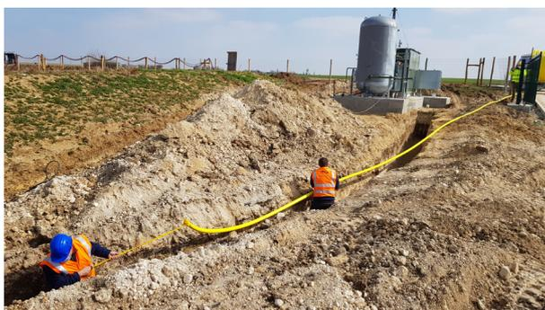
The pipe is completely constructed from advanced polymers and rules out time consuming welds and the associated x-ray tests. Pipe corrosion is also a problem of the past.
